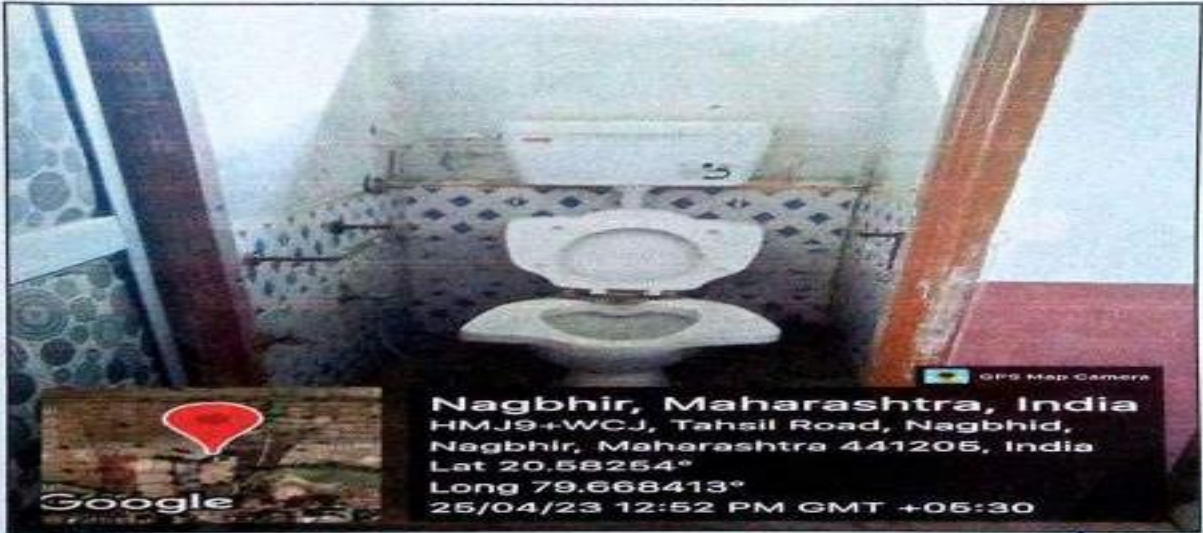
7.1.7 DISABLED FRIENDLY WASHROOM
