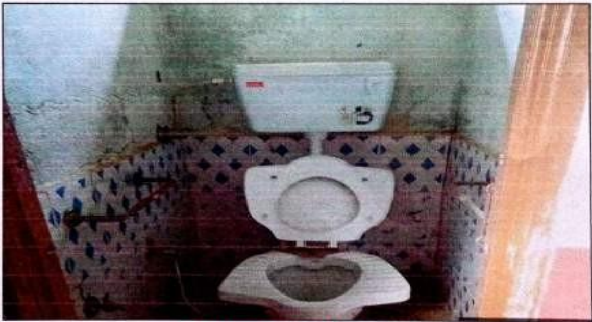
7.1.7 DISABLED FRIENDLY WASHROOM
