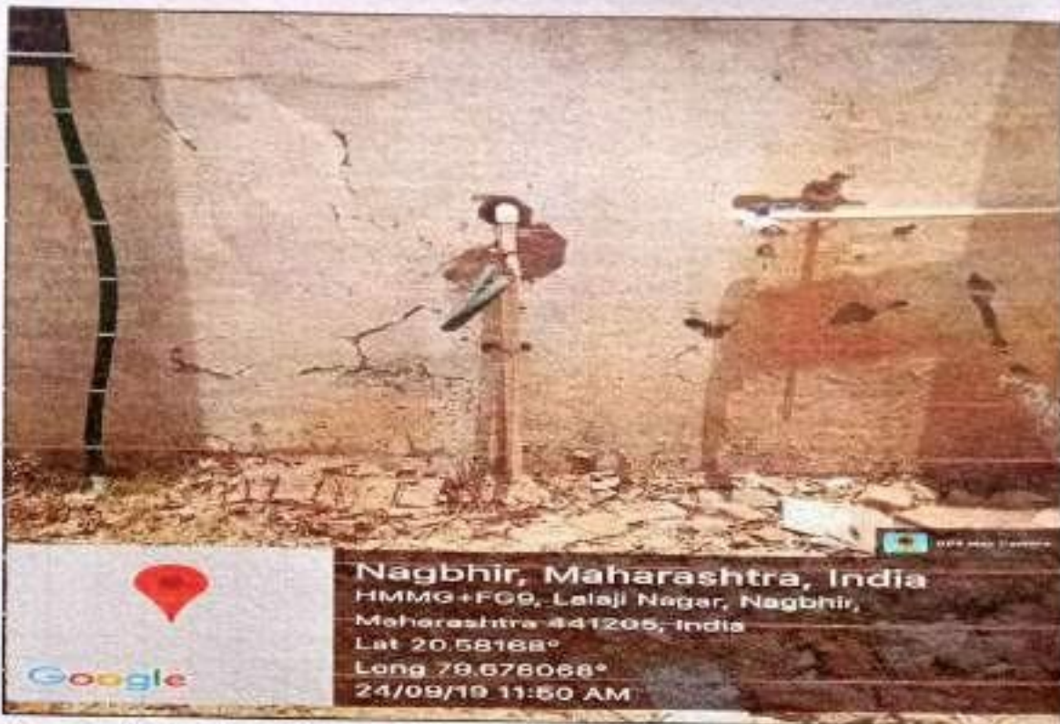
7.1.4 RAIN WATER HARVESTING
