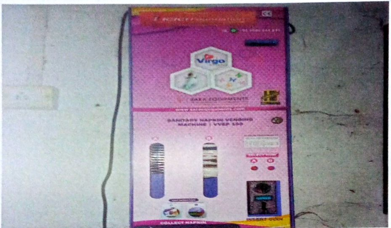
AUTOMATIC VENDING MACHINE INSTALLATION OF IN THE GIRLS COMMON ROOM.
